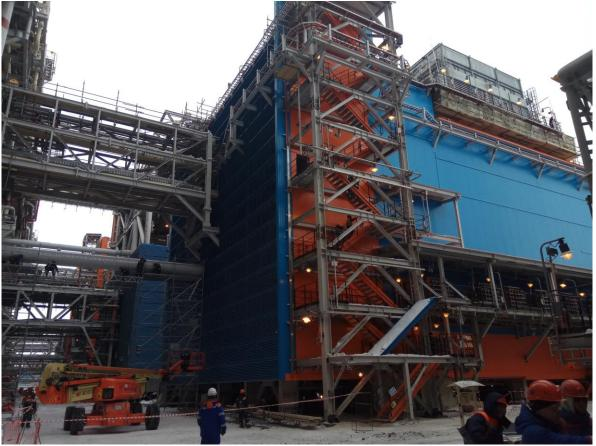
FIRETEX M90 series is an epoxy thick layer coating, provides up to 240 minutes hydrocarbon pool and jet fire protection. The material has high chemical resistance, it can be used at operating temperatures as low as -60°C and as high as +75°C, which allows its use under conditions of an open industrial atmosphere of a cold climate.
